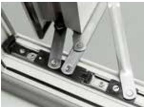
The sliding track on friction hinges must not be lubricated. The amount of friction on the hinge can be adjusted by turning the adjusting screw.
