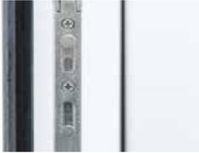
Periodic lubrication of the espagnolette locking system with a light acid-free lubricant will help to ensure a smooth operation. Strikers are 'mushroom' shaped and can be turned using an Allen key. Take care not to adjust the strikers to require too much pressure as this will strain the espagnolette. It should be possible to comfortably turn the handle when closing the window without having to force it.
