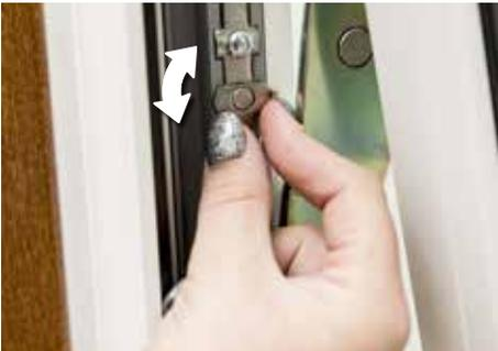
As a child safety device, the restrictor can be locked in any of its set opening positions. To lock the restrictor turn the disc plate on the hinge a quarter turn clockwise. To release the restrictor, turn the disc plate on the hinge a quarter turn anti clockwise.
