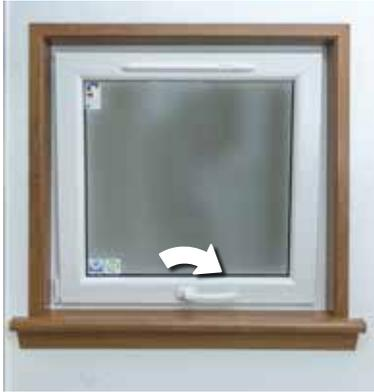
Opening the window into the tilt (ventilation) position
